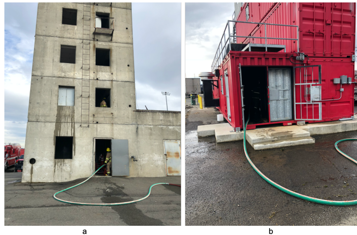
Figure 4. (a) Photo of concrete building used for live-fire experiments with Fire Department teams. (b) The second building was composed of multiple stacked corrugated metal shipping containers.
